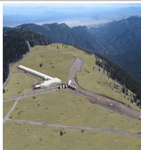
MROI - Magdalena Ridge, NM (under construction)
