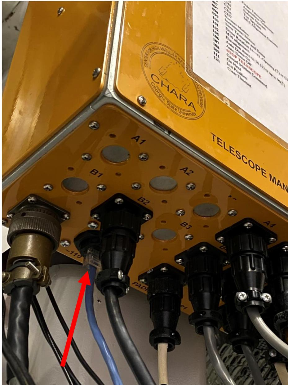
Unplug the cable, wait a second or two, and plug it back in. Restart the HuT server in the usual way and communications should be restored. Looking at the indicator light on the right side of the TEMA box again, the top indicator LED should now be lit green as pictured. Confirm that the HuT is back up and running by moving something, Fiber Lid, Corner Cube, etc.
